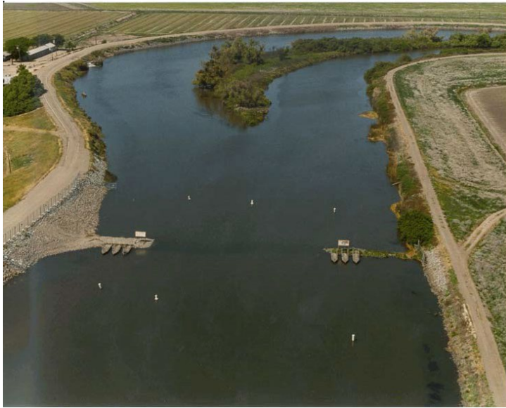
Figure 3. Middle River Barrier Weir (central weir not visible due to overtopping)
