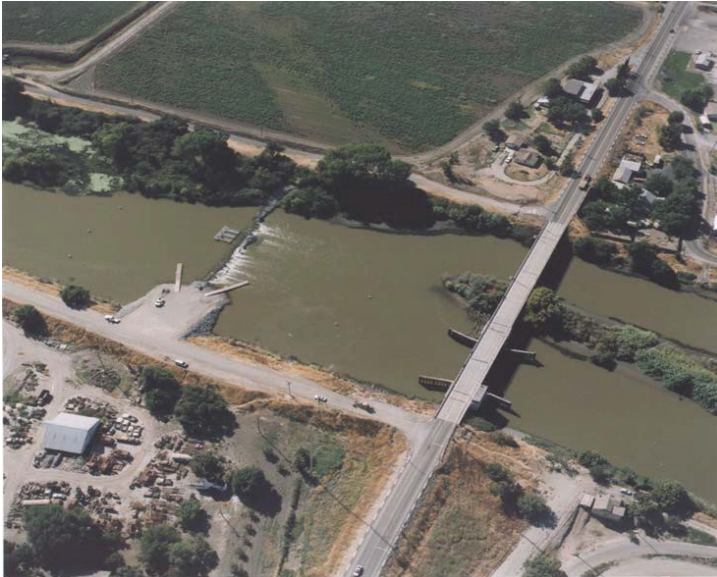
Figure 5. Grant Line Canal Barrier
